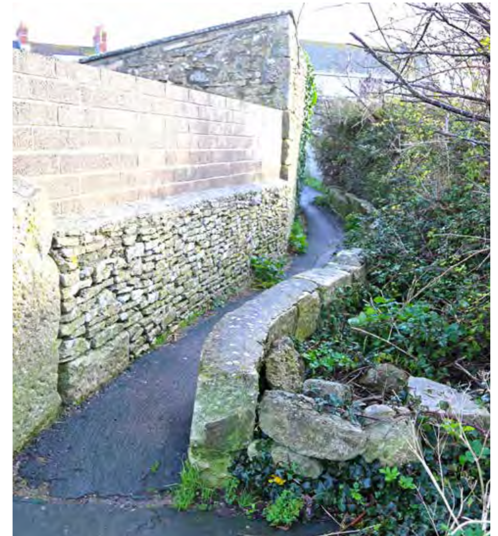
PRoW from Rip Croft to Avalanche Road
