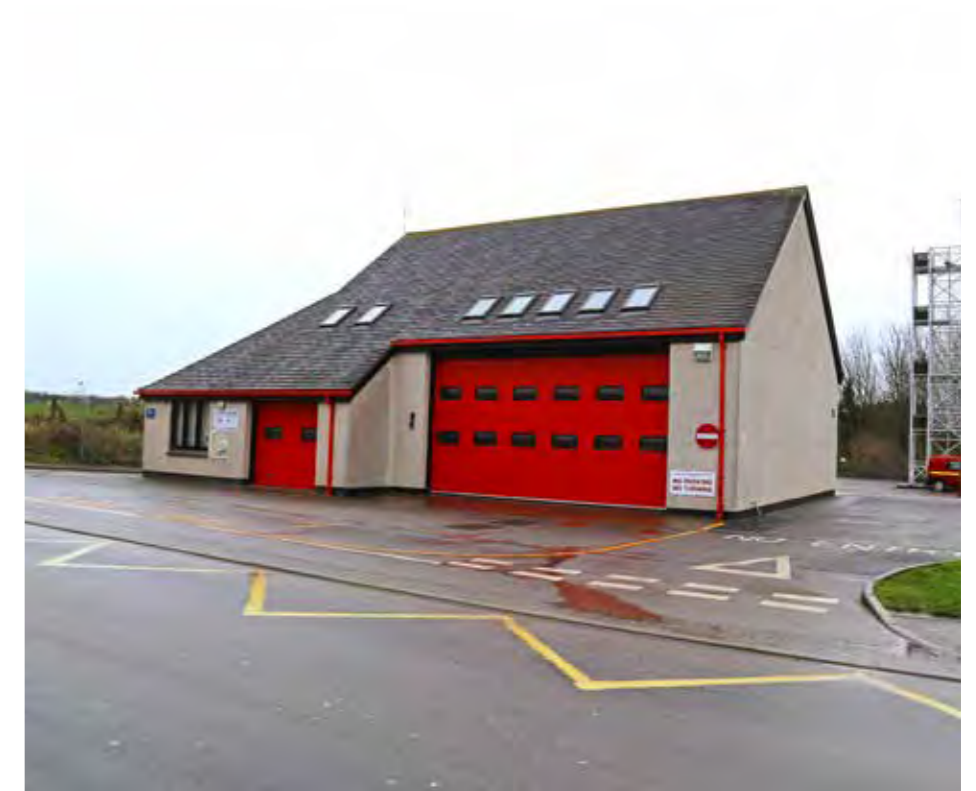
Portland Fire Station and Police Station
